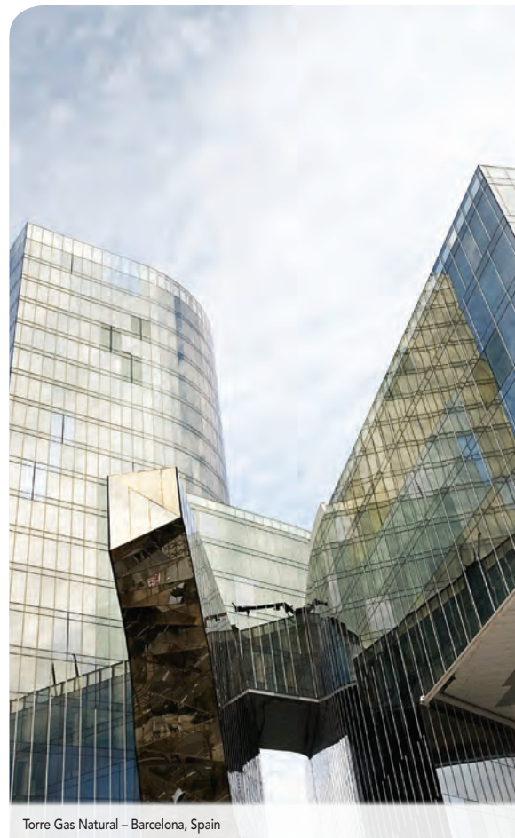
Torre Gas Natural – Barcelona, Spain
